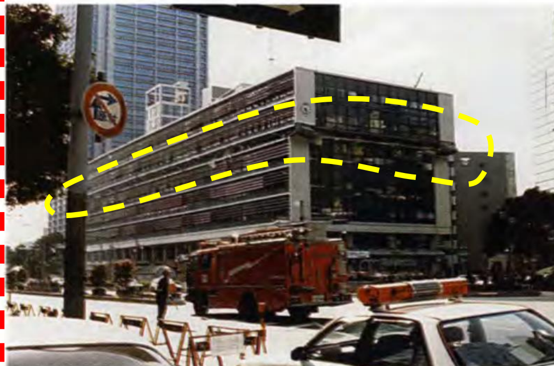
Fig. 20. Kobe City Hall, which collapsed at the sixth floor.
